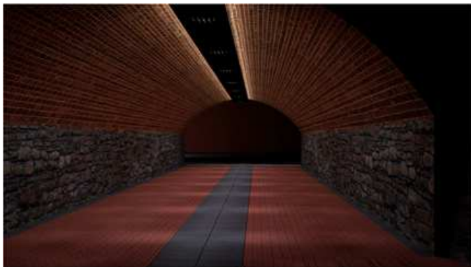
Paxton Tunnel lighting feature
